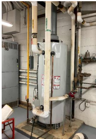
DHW Heater: Core Building
