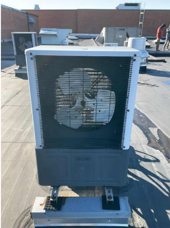
Condensing Unit-Rooftop
