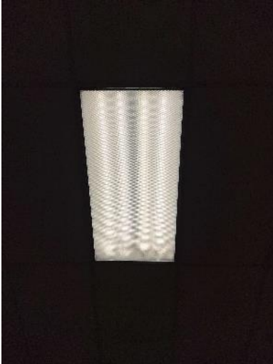
Linear Fluorescent T8 Fixture
