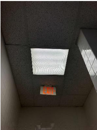
U-Bend Fluorescent T8 Fixture
