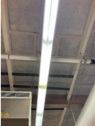
Linear Fluorescent T8 Fixture
