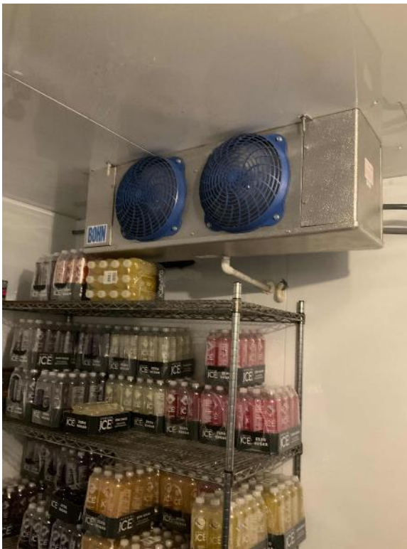
Walk-in Cooler: Exterior: 9/10 Building
