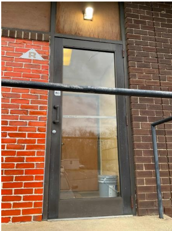
Doors: Warehouse Entrance
