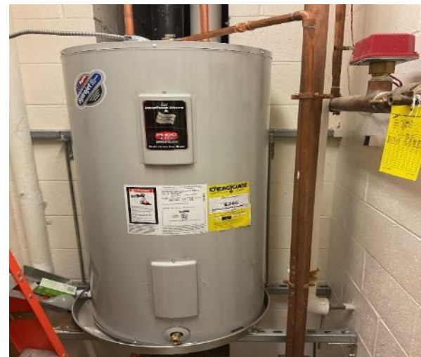
Typical Electric Hot Water Heater
