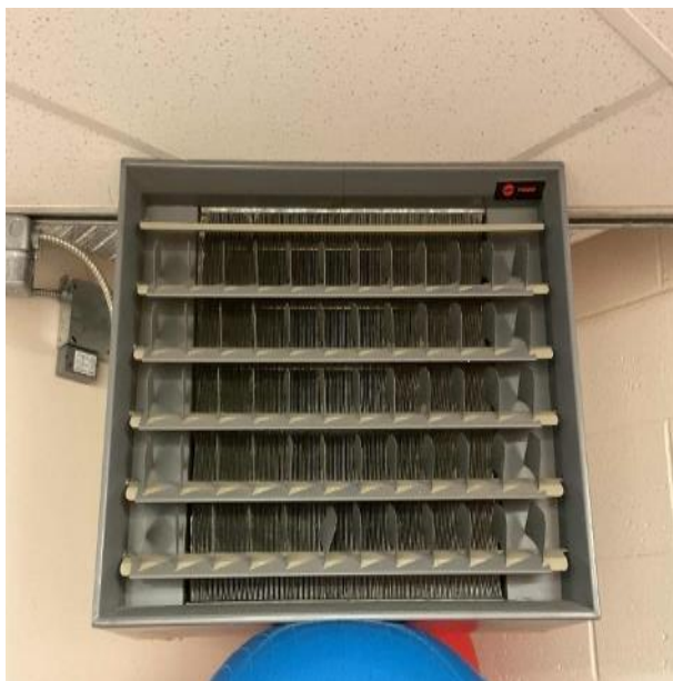
Typical Hydronic Unit Heater
