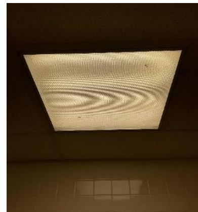
T8 U-bend Linear Fluorescent Fixtures
