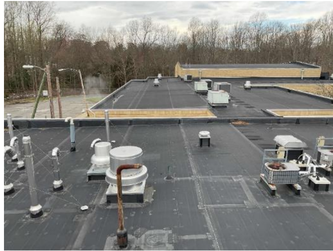
Flat Roof with Black Membrane
