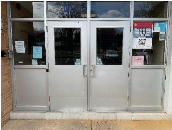
Main Entry Door
