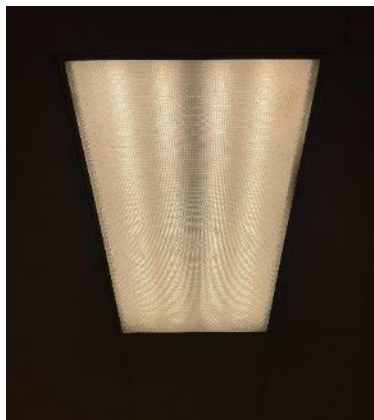
T8 U-bend Linear Fluorescent Fixtures
