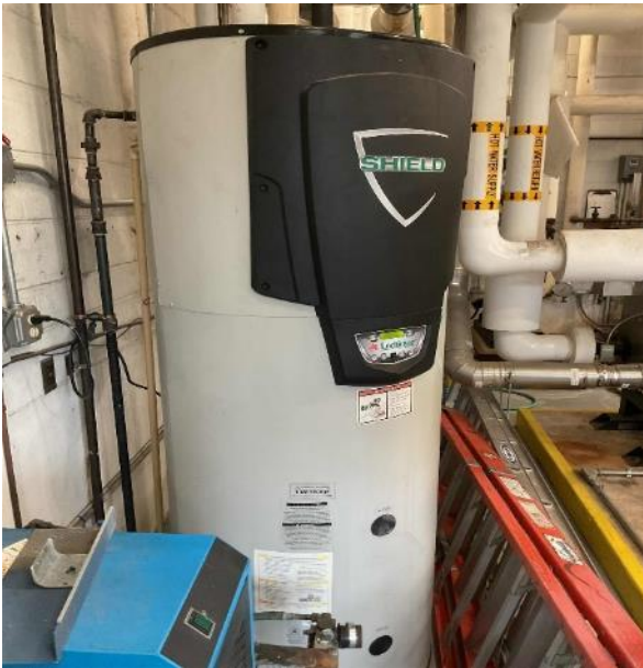
Lochinvar Natural Gas Hot Water Heater
