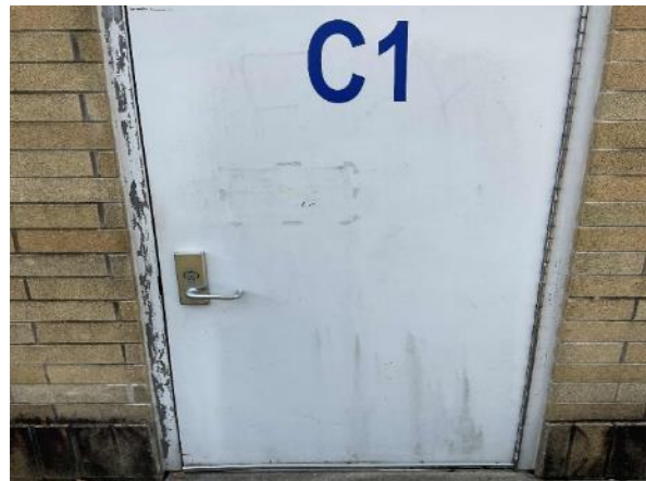
Typical Exterior Doors
