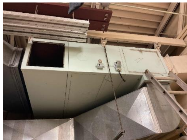
Unlabeled AHUs in Ceiling of Stage Area
