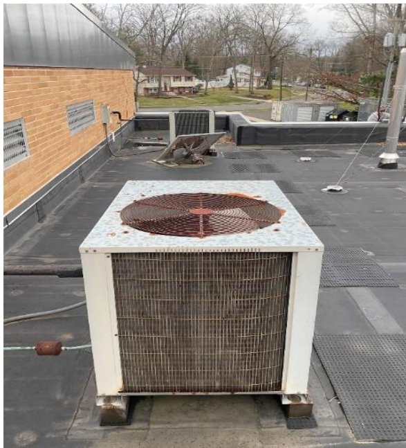
Condensing Units Serving Air Handler
