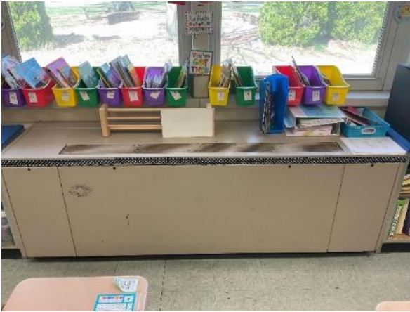
Typical Classroom/Office Unit Ventilator
