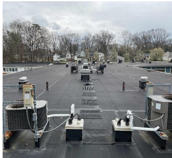
Condensing Units Tied to Unit Ventilators
