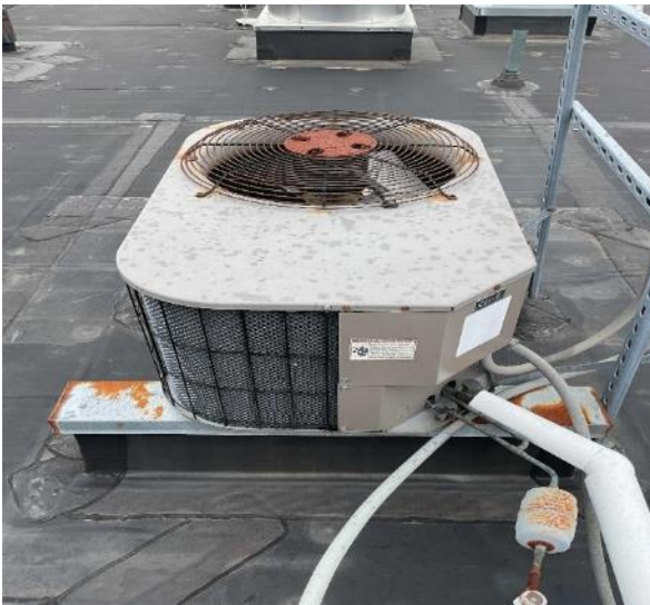
Condensing Units Tied to Unit Ventilators
