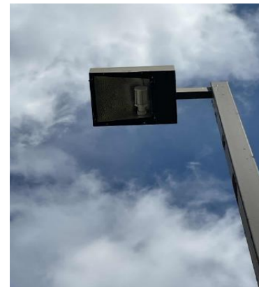
LED "Corn bulb" Retrofit in Parking Lot Lighting
