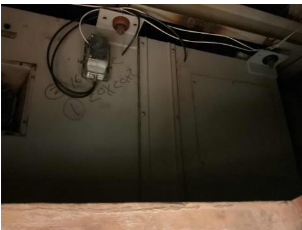
Unlabeled AHUs in Ceiling of Stage Area
