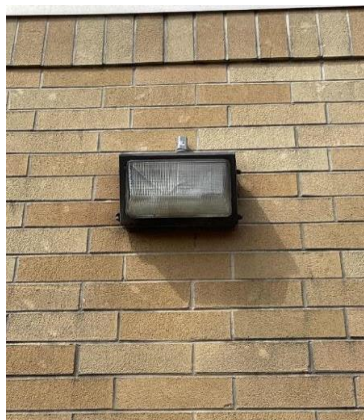
Typical Exterior LED Wall Pack and Metal Halide Lights
