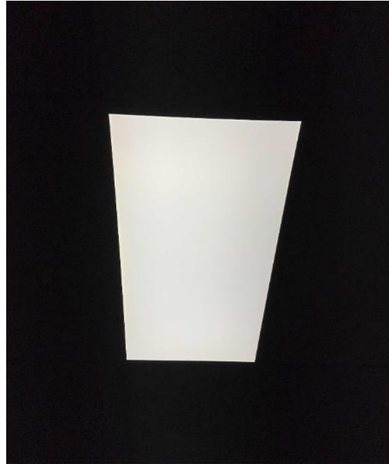
LED 2-foot x 4-foot Fixture-Conference Room
