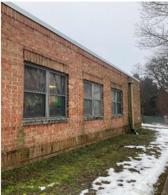
Back Side- Building Envelope
