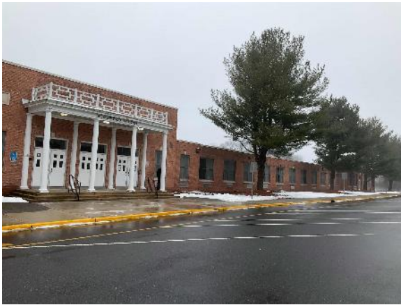
Front Side- Building Envelope
