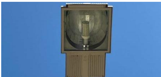
Exterior LED "Corn" Bulb- Pole Mounted
