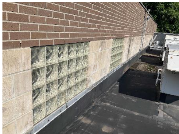
Building Envelope- Roof View
