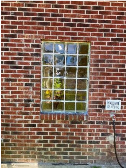
Window and Brick Façade at Hawkins
