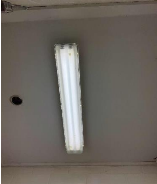
Linear Fluorescent T8 fixture at Conover Hills
