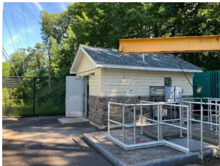
Stone and Vinyl Siding at Greenwood Road
