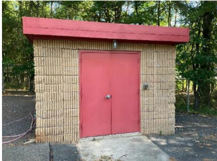
Brick Façade at Millponds
