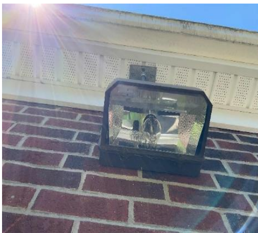
Metal Halide Wall Pack at Hawkins
