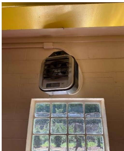
5 kW Unit Heater at Hawkins
