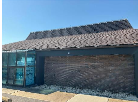
Building Envelope: Old Admin Building
