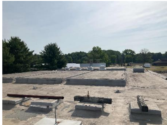
Building Roof: Filter Building
