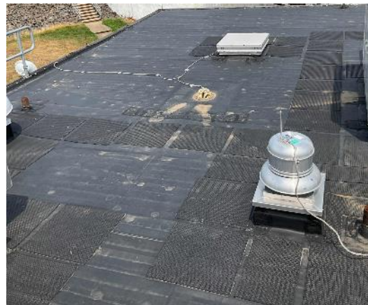
Building Roof: Pump Station
