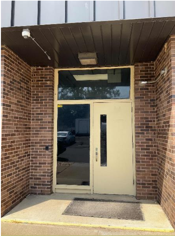
Building Door: Nitrification Building
