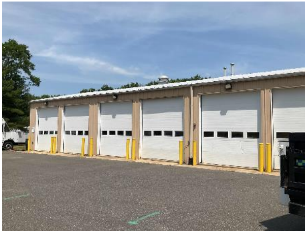
Building Envelope: Collection Vehicle Garage
