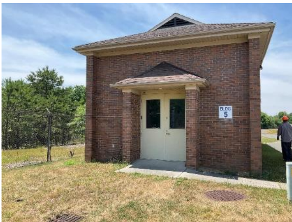
Building Envelope: Pump Station Control
