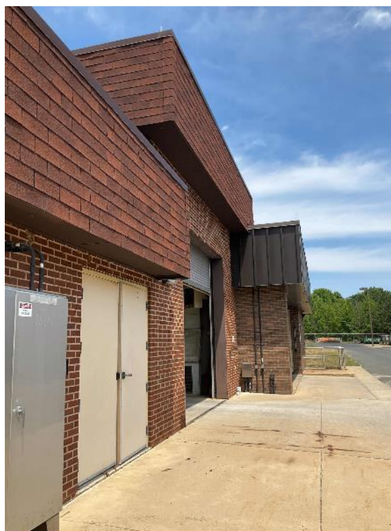
Building Envelope: Pump Station
