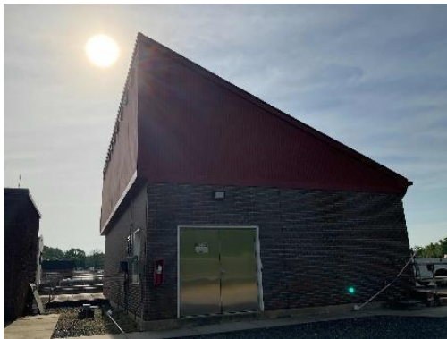
Building Envelope: U.V. Disinfection
