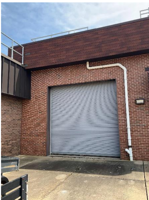
Overhead Door: Pump Station
