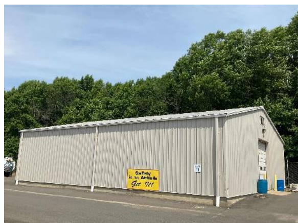
Building Envelope: Plant Storage
