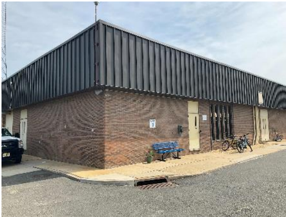
Building Envelope: Filter Building
