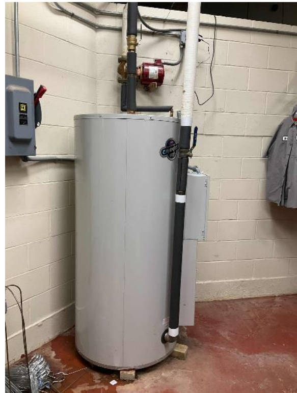
Electric Storage Water Heater: FMB
