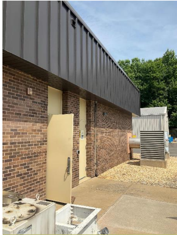
Building Envelope: Nitrification Building
