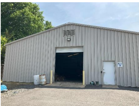
Building Envelope: Plant Storage
