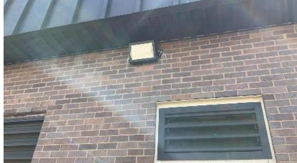
Exterior LED Wall Pack: FMB
