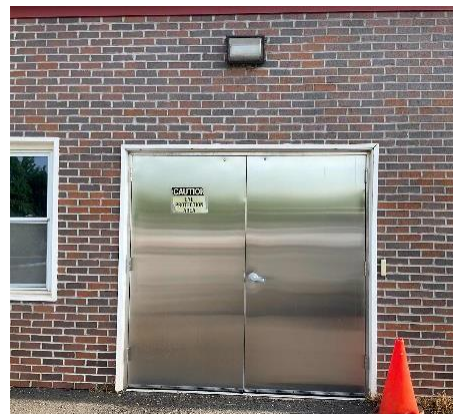
Building Door: U.V. Disinfection
