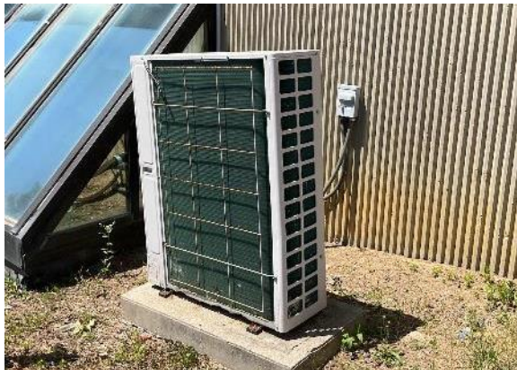
Split Condensing Unit: FMB
