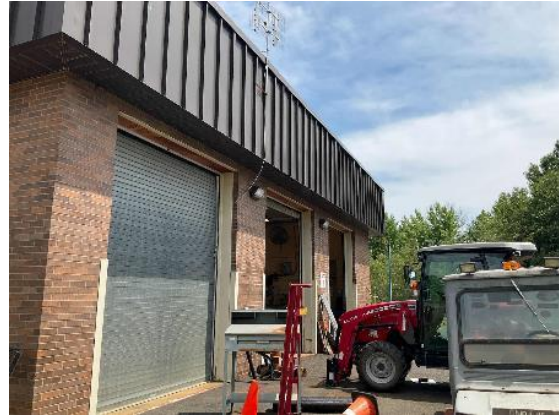
Building Envelope: Plant Maintenance Garage
