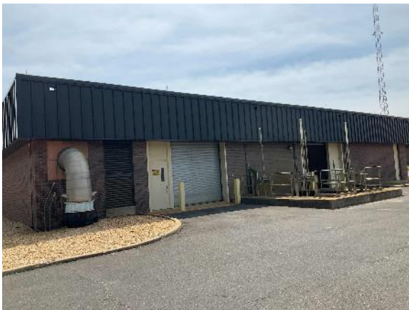
Building Envelope: Nitrification Building
