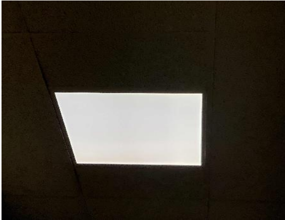
LED 2-foot x 2-foot Fixture: Filter Building
