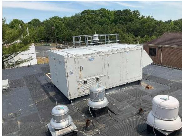
Exhaust Fan: Pump Stations
