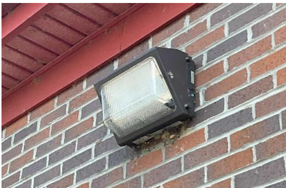
Exterior LED Wall Pack: U.V. Disinfection
