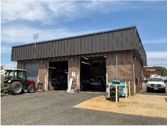
Building Envelope: Plant Maintenance Garage
