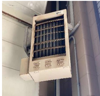
Manual Dial Thermostat: Pump Station
