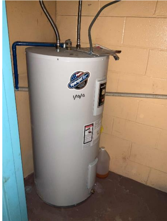
Electric Storage Water Heater: Pump Station
