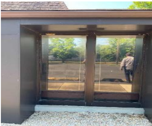
Building Door: Old Admin Building
