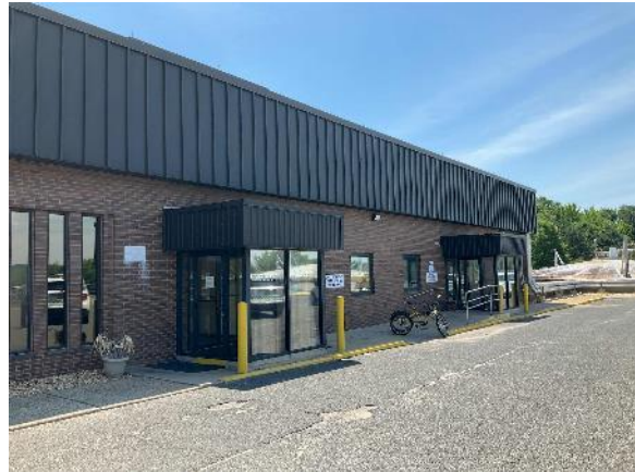
Building Envelope: FMB
