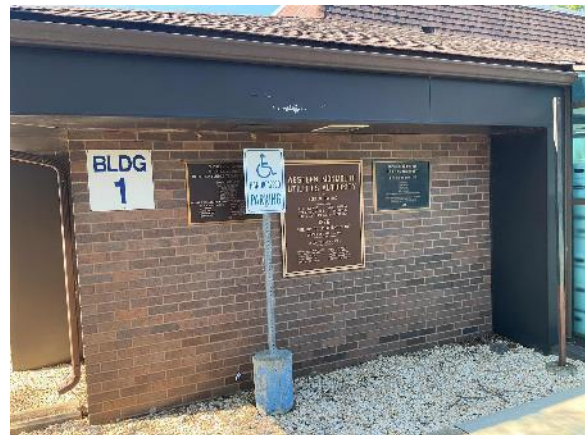
Building Envelope: Old Admin Building
