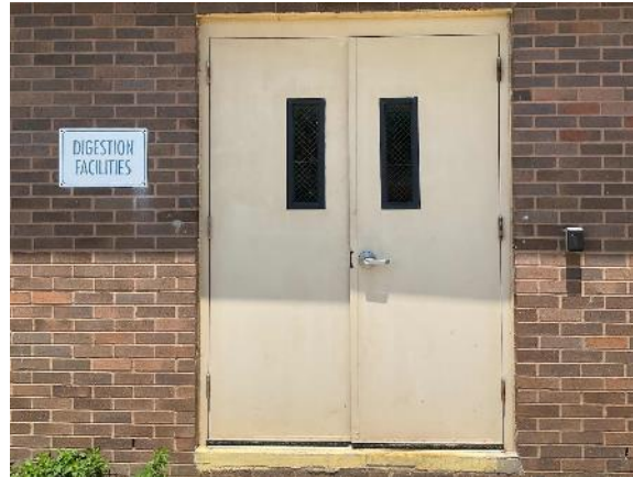
Building Door: Digester Building
