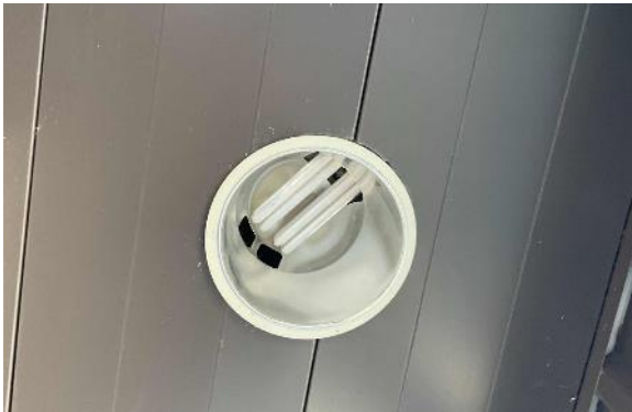
Exterior CFL Can Fixture
