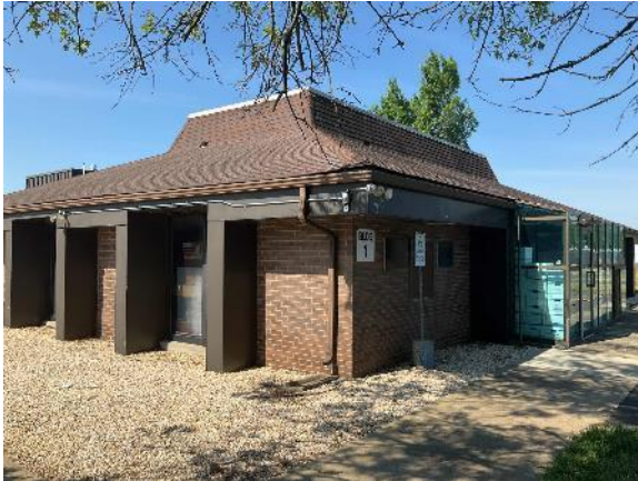
Building Envelope: Old Admin Building
