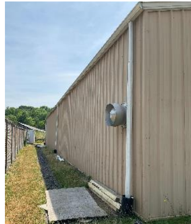
Building Envelope: Collection Vehicle Garage
