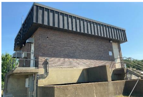
Building Envelope: Grit Building
