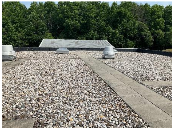
Building Roof: Nitrification Building
