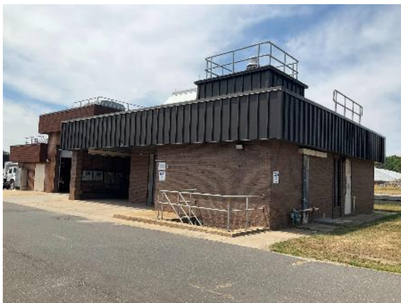
Building Envelope: Pump Station
