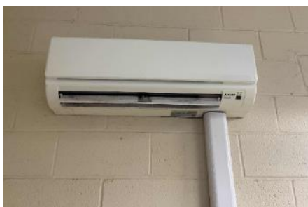
Wall-Mounted Indoor Unit: Pump Station Control
