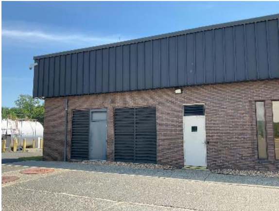
Building Envelope: FMB
