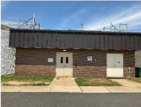
Building Envelope: Digester Building
