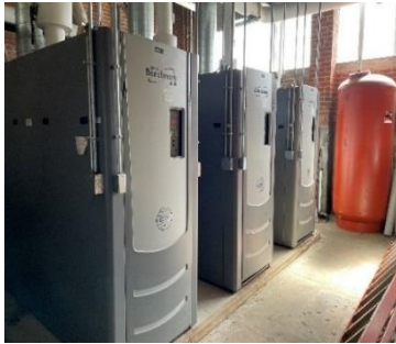
AERCO Condensing Hot Water Boiler
