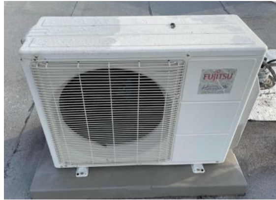
Split air source Heat pump
