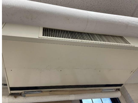
Ceiling-mounted Unit Ventilator
