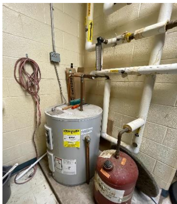
Electric DHW Heater
