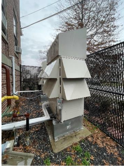
VRF Ductless Mini-Split HPs
