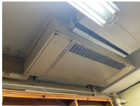
Ceiling Mounted Unit Ventilator
