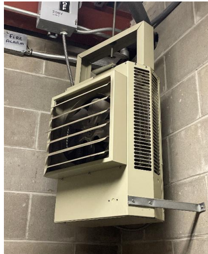
Electric Unit Heater
