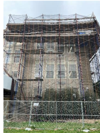
Exterior Under Construction Roof
