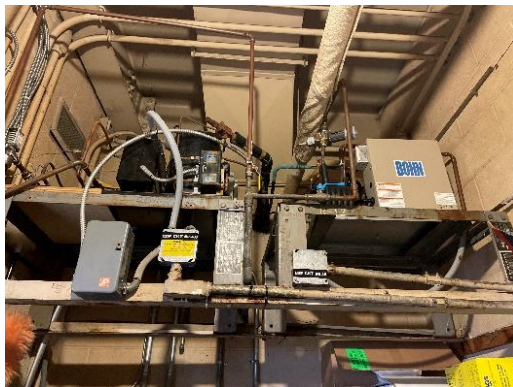
Walk-in Compressors
