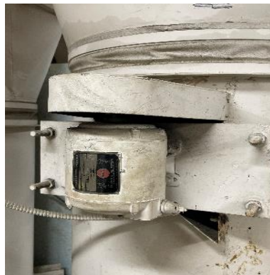
AHU Motor
