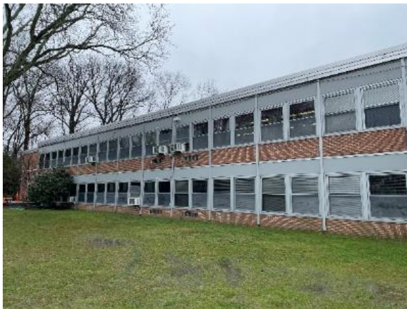
Side of Building
