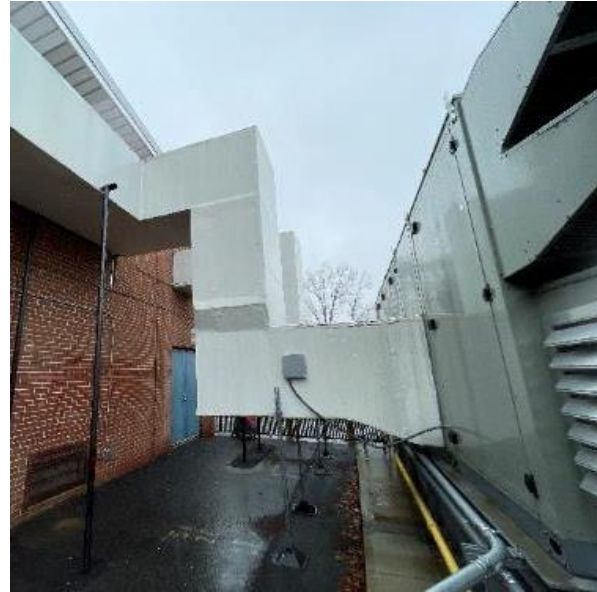
RTU Ducting
