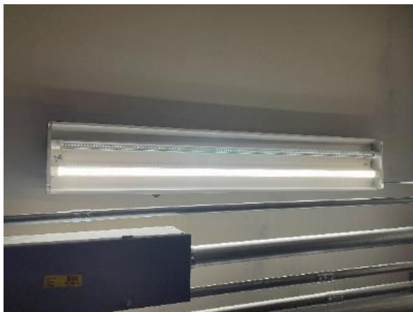
Surface Mounted Linear Tube LED
