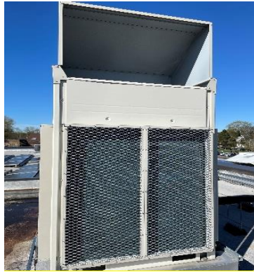
10 Ton Ductless Mini-Split HP
