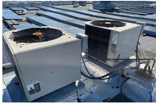
Split DX Condensing Units
