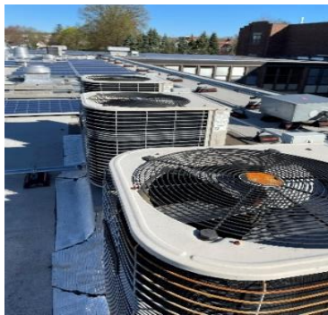
Split DX Condensing Units
