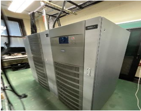
CRAC Indoor Unit
