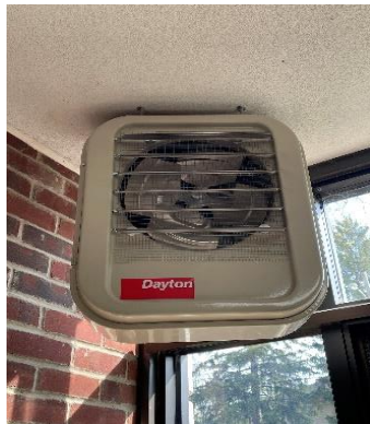
Electric Unit Heater
