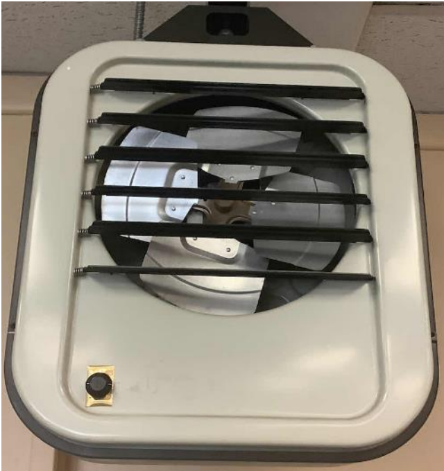
Electric Resistance Heaters
