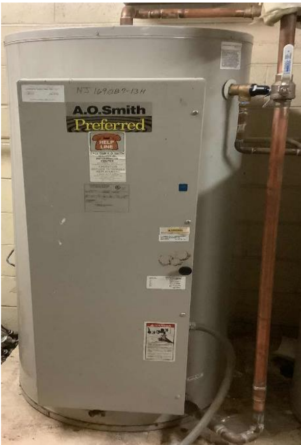
Electric Storage Tank Water Heaters
