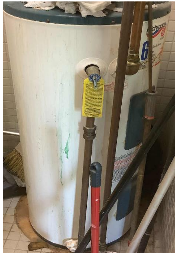
Electric Storage Tank Water Heaters
