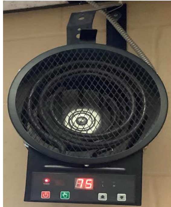
Electric Resistance Heaters
