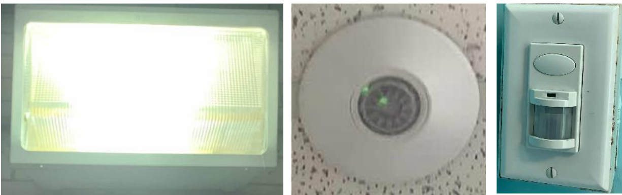
Natatorium High Pressure Sodium Fixture & Occupancy Sensors
