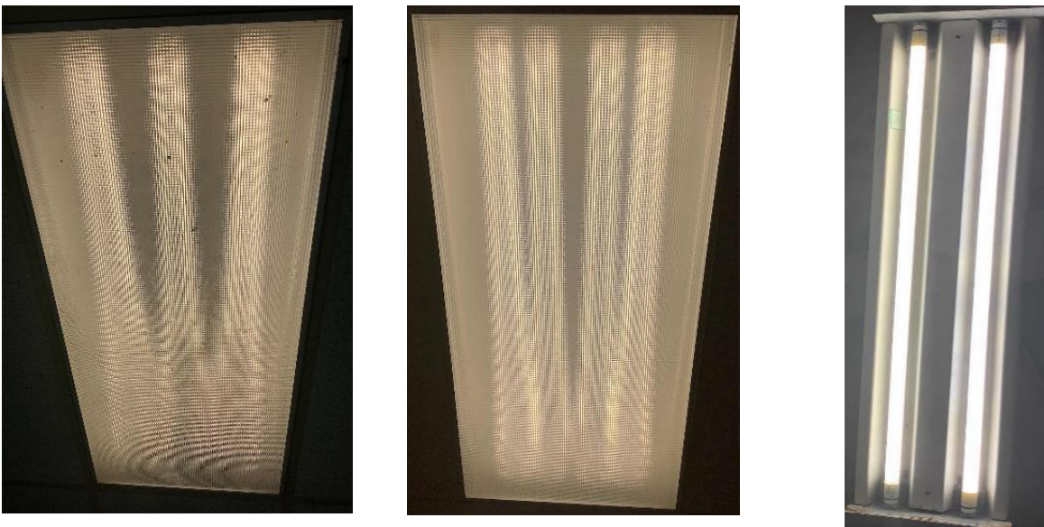
Linear Fluorescent T8 and LED Fixtures
