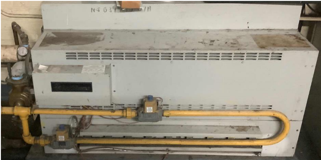
Gas-fired Domestic Hot Water Boiler
