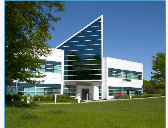
The Colgate-Palmolive Global Technology Center received a combination of prescriptive and custom SmartStart incentives to help offset the cost of installing more energy-efficient chilled water plants.
