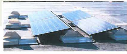
2 TYPICAL BALLASTED SOLAR RACKING SYSTEM PV1.0 SCALE: 1/8"
