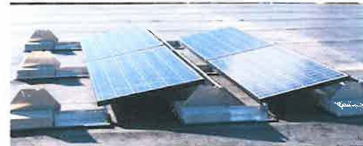
2 TYPICAL BALLASTED SOLAR RACKING SYSTEM SCALE SITE
