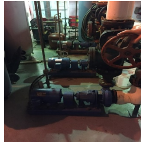
Heating Hot Water Pumps
