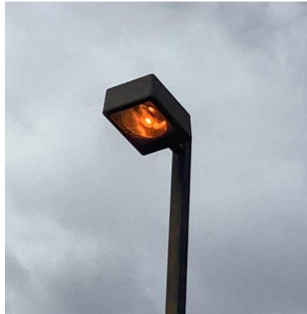
Exterior HPS Fixtures
