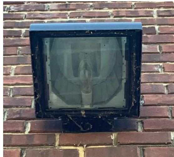
Exterior HPS Fixture
