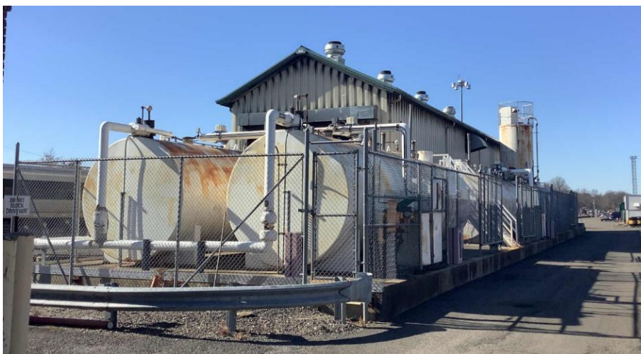
Diesel Fuel Tanks
