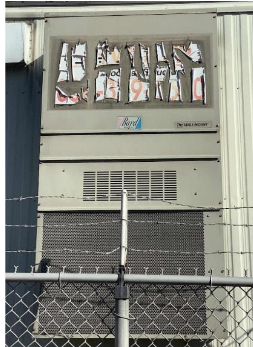
Through-the-Wall AC Units
