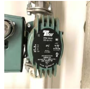
DHW Recirculation Pump
