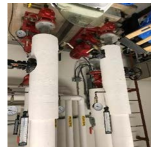
Heating HW pumps
