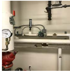
DHW Pipe Insulation
