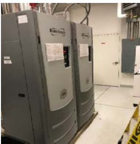
Condensing Boilers
