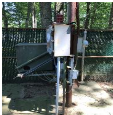
Wire Mesh Structure
