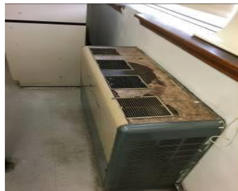
Image 6 – Unit Ventilator
