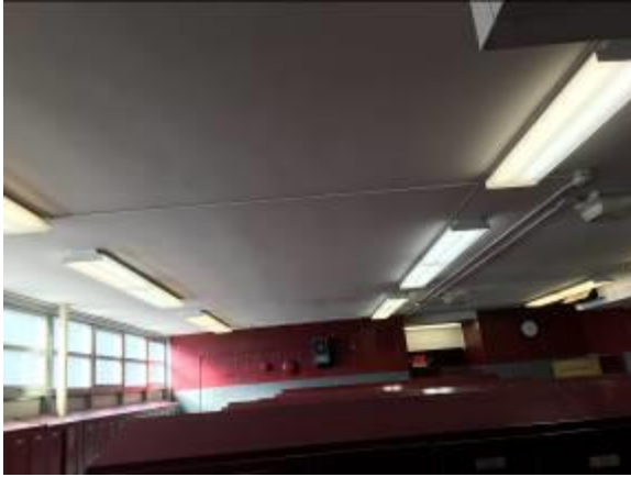
Image 3 – T8 Fluorescent Lighting (locker room)
