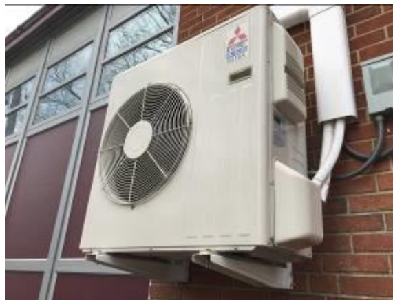
Image 8 – Split HP Outdoor Coil Unit (Server Room)
