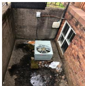
Outdoor Condensing Unit for Split AC System
