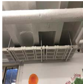
Steam Radiator with Manual Dial Valve
