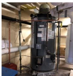
Storage Tank Water Heater
