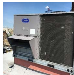
Packaged Roof Top Unit
