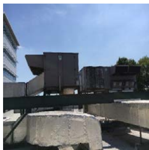
Packaged Roof Top Units
