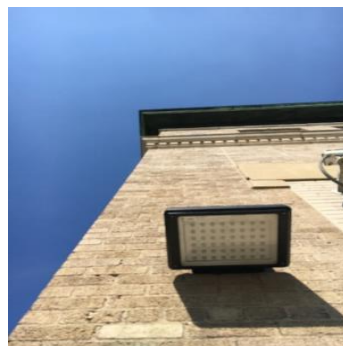
Wall-Mount LED Fixture
