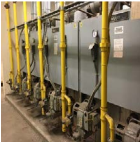
Hydrotherm Hot Water Boilers
