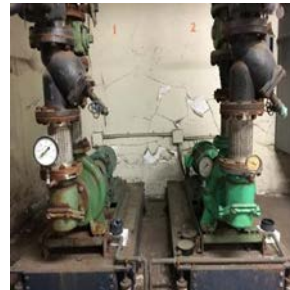
Heating Hot Water Pumps
