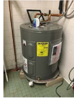
DHW Tank for Slop Sink
