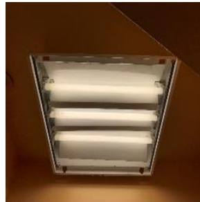
Linear Fluorescent Fixture No Lens
