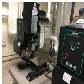
Condensing Hot Water Boilers
