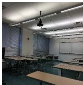
Pendant-mounted Linear Fluorescent Fixtures
