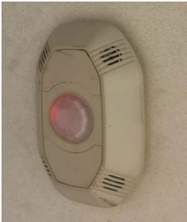
Ceiling Mounted Occupancy Sensor
