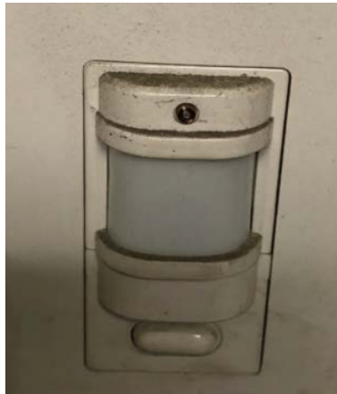
Wall Mounted Occupancy Sensor
