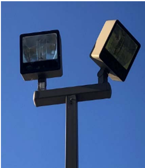
Pole Mounted HID Fixture
