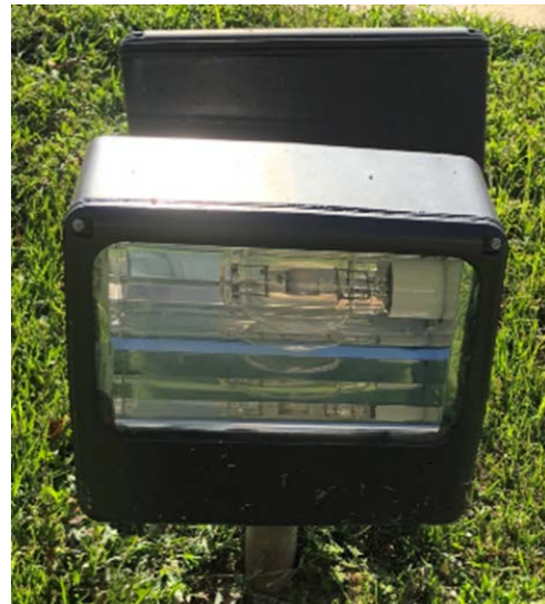
Ground Mounted HID Fixture
