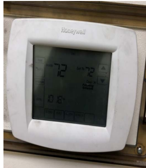
PTHP & Programmable Thermostat
