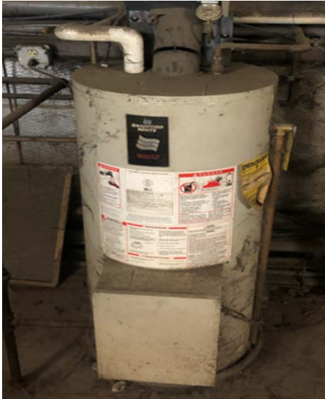
38 Gallon Gas-Fired & 19 Gallon Electric Water Heaters
