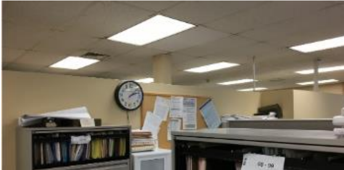
Interior 4' 2-Lamp T8 Fluorescent Fixtures
