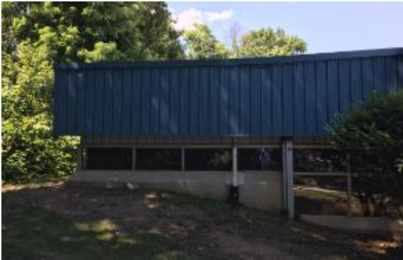
Exterior Wall and Windows
