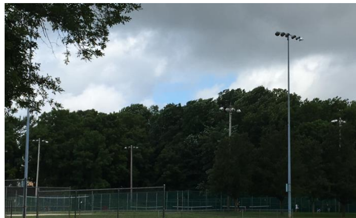
Field and court lights
