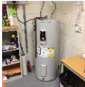
Figure 11 - Domestic Hot Water Heater
