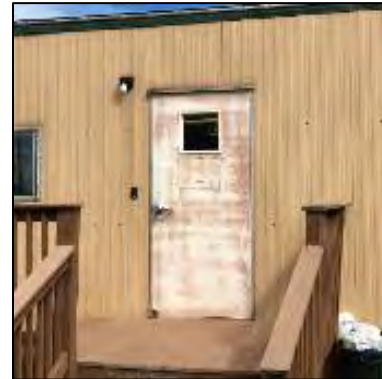
Picture 4: Exterior doors
