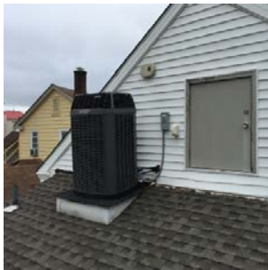
Exterior Walls and Roof
