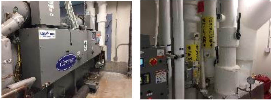
Figure 12 – WSHP Equipment
