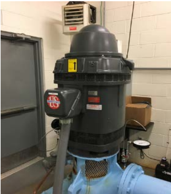
100 hp Well Pump Motor
