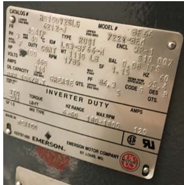
100 hp Well Pump Motor
