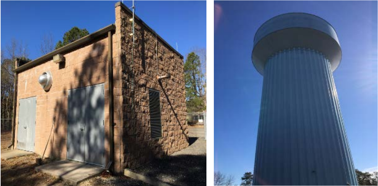
Well Building & Elevated Water Storage Tank
