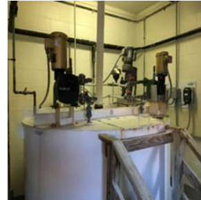
Lime & Mixing Pumps
