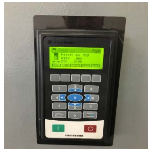
Variable Speed Drives (VFDs)
