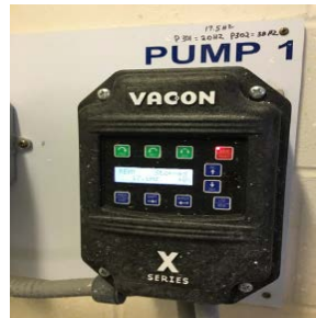
Variable Speed Drives (VFDs)
