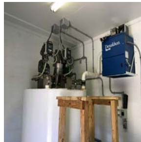
Lime, Mixing Pumps and Variable Speed Drive (VFD)
