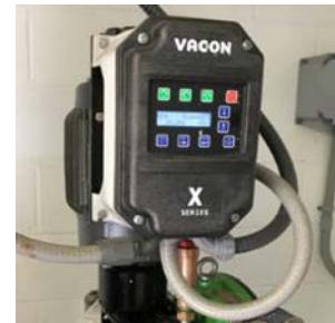
Lime, Mixing Pumps and Variable Speed Drive (VFD)
