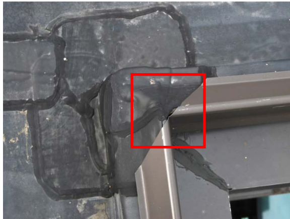
Aluminum Corner Flashing/ EPDM Detail
