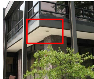
Exposed Second Floor Area
