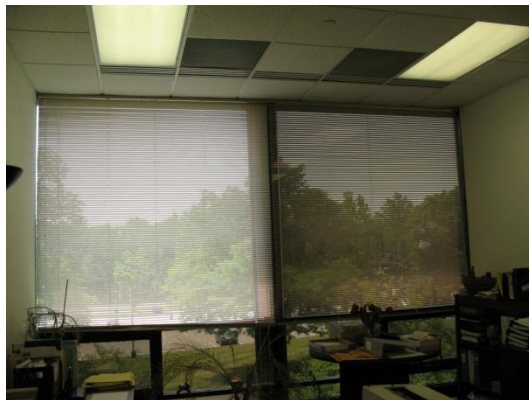
Single Pane Windows on 2 nd floor – left window missing film Some 2 nd Floor Windows Missing Window Film
