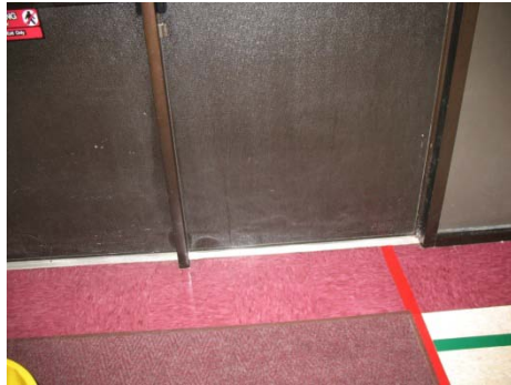
Double doors in good condition
