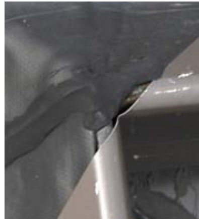
Close-Up View Shows Leak
