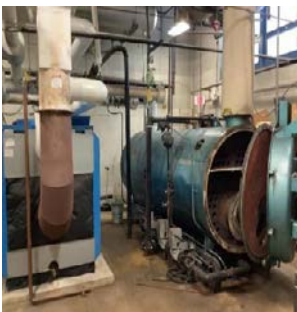
Non-Condensing Hot Water Boilers
