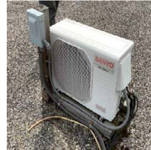
Ductless Mini-Split System AC
