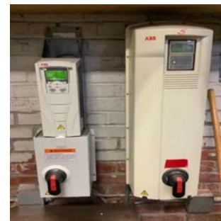
Hot Water Pump VFDs
