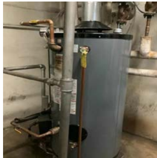
Gas-Fired Storage Water Heater
