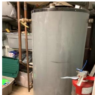
Gas-fired storage water heater
