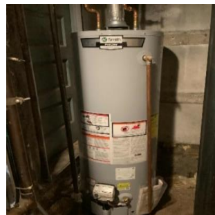
Domestic hot water heater
