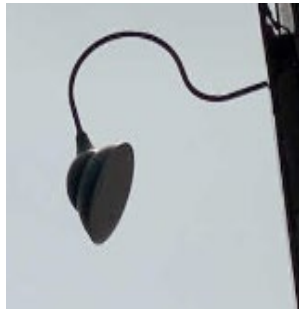
Sign lighting Controlled by Wall Switch
