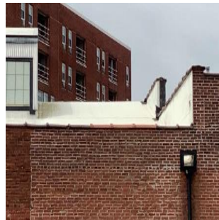
White EPDM Roofing
