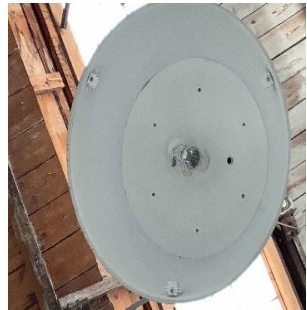
Interior High Bay lighting
