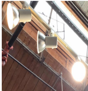
Presentation Lighting Control
