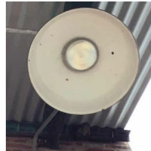
Sign lighting controlled by wall switch
