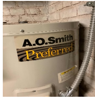
Electric Storage Tank Hot Water Heater
