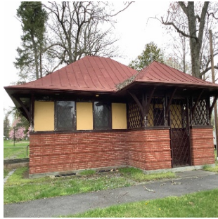
Exterior of Building
