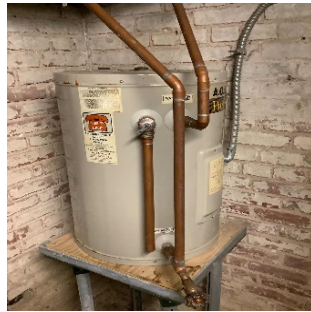
Electric Storage Tank Hot Water Heater
