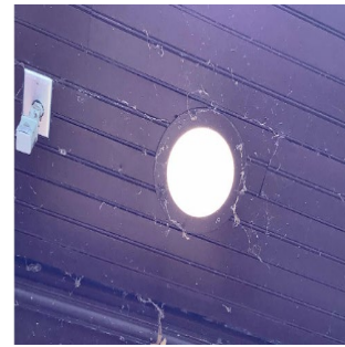
Exterior Canopy Fixture
