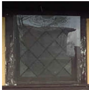
Window with Plexiglass Covering
