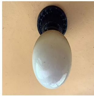
Interior LED Fixture
