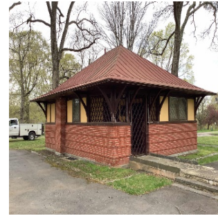
Exterior of Building
