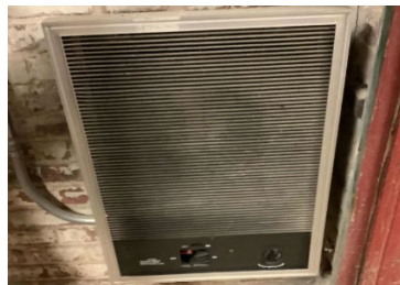
Basement Electric Resistance Heater
