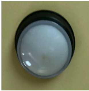
Interior LED Fixture
