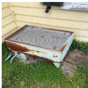
Outdoor Condensing Unit
