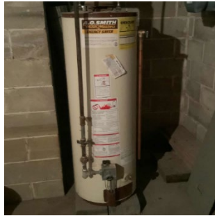
Gas-Storage Hot Water Heater
