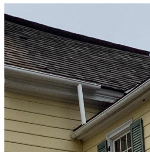
Roof - Wood Shingles
