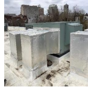
Roof Top Units (RTUs)
