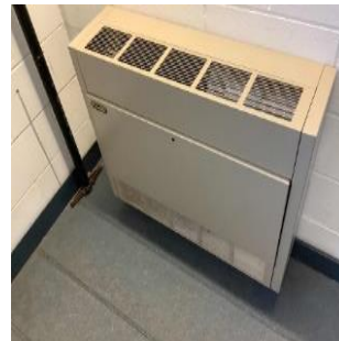
Electric Resistance Heater
