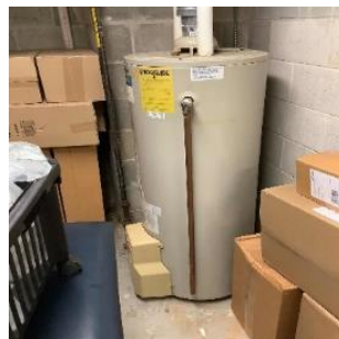
Gas-fired Storage Water Heater
