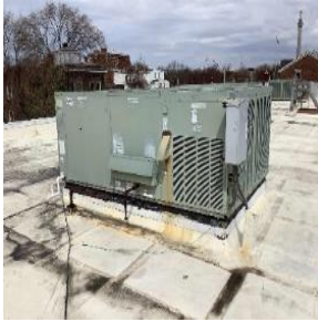
Roof Top Units (RTUs)
