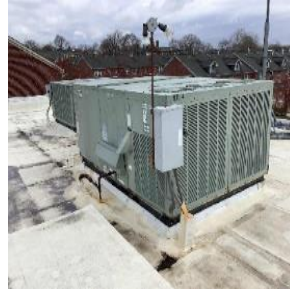
Roof Top Units (RTUs)
