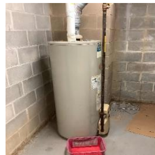
Gas-fired Storage Water Heater
