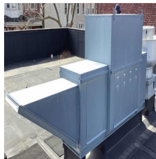
Kitchen Make-Up Air Unit
