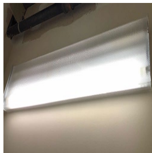
Linear Fluorescent Fixture
