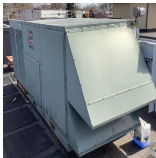
Rheem Gas-Fired Packaged RTU
