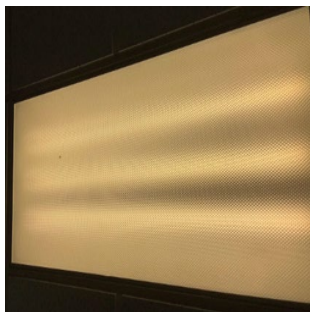
Linear Fluorescent Fixture
