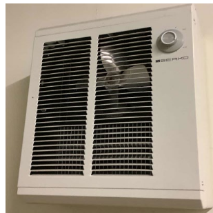
Electric Resistance Heater
