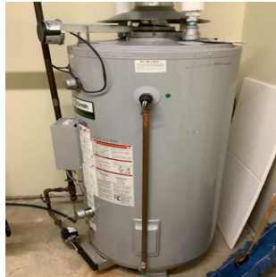
Gas-Fired Storage Tank Water Heater
