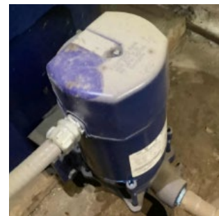
Feed Water Pump
