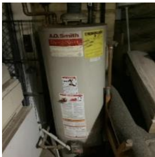
Domestic Hot Water Heater
