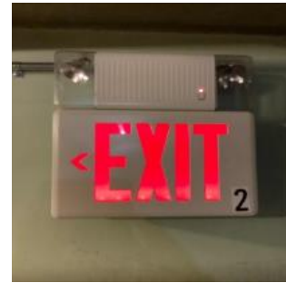
LED Exit Sign
