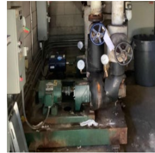
Chilled Water Pumps
