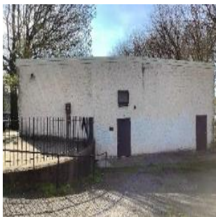
Exterior of building
