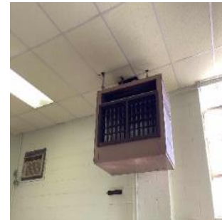
Hanging Gas-fired Furnace,
