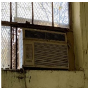
Window AC Units
