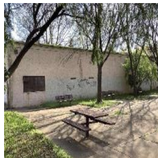
Exterior of building
