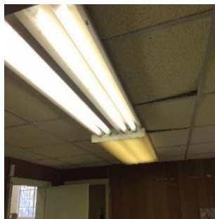
Surface Mount Wrap Fixtures in Office
