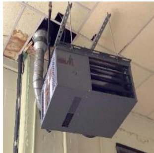
Hanging Gas-fired Furnace
